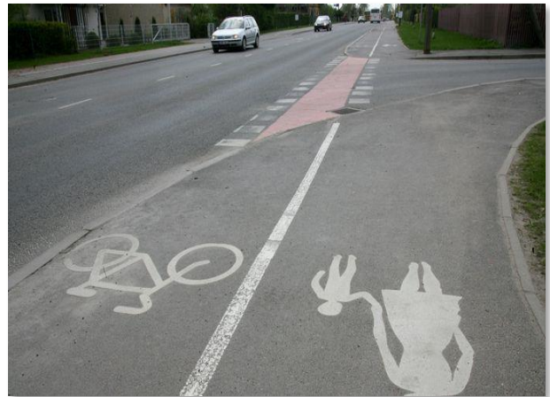
Picture 1. Comparison of the road surface marking of current combined traffic (on the left) and road surface marking of planned separated lanes (on the right).
